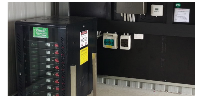
Rack-mounted lithium battery
